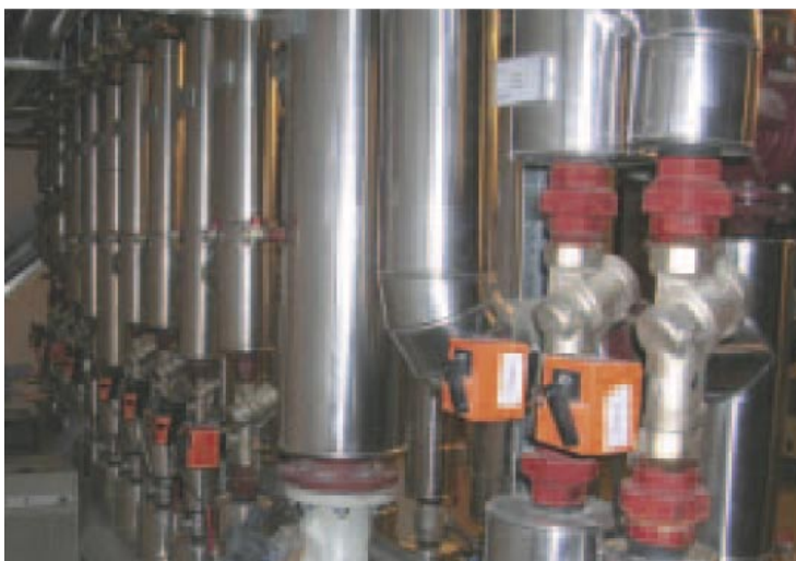
Hydraulic balancing is no longer necessary with the pressure-independent characterised control valves and globe valves from Belimo, which saves on time, costs and nerves.
