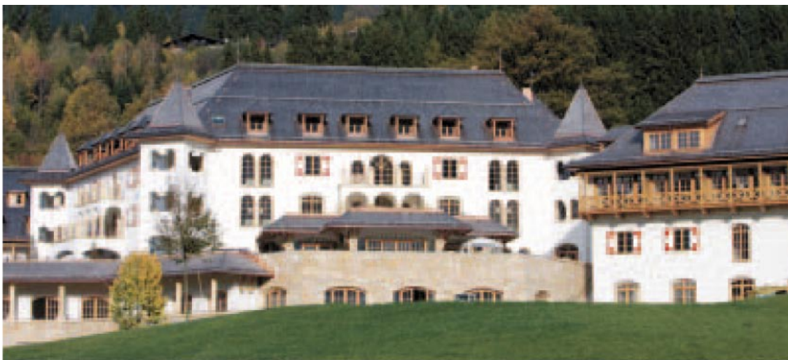
The architecture of the new Grand SPA Resort A-ROSA in Kitzbühel fits perfectly into the surroundings and was built in the style of a Tyrolian castle.
